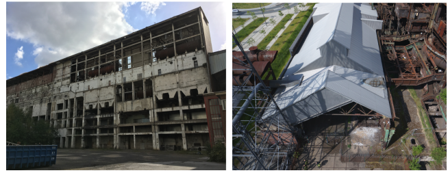
Figure 13. Buildings of the Gustav Knepper powerplant (left) and the Phoenix-West foundry (right).
