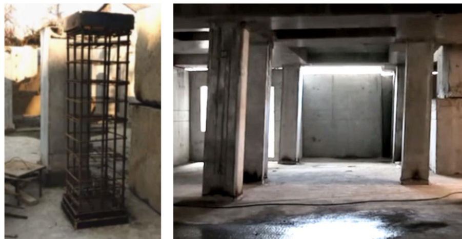
Figure 2. Rocking columns in bottom ‘kinematic bearing’ story: completed and unfinished column [14] (left) and initial displacement of the ‘kinematic bearing’ story in a free-rocking-motion test [15] (right).
