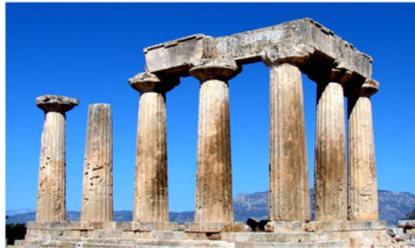
Figure 3. View of the Temple of Apollo, in Corinth, Greece. Its monolithic, free-standing columns support massive epistyles and remain standing in an area of high seismicity since 540 BC.
