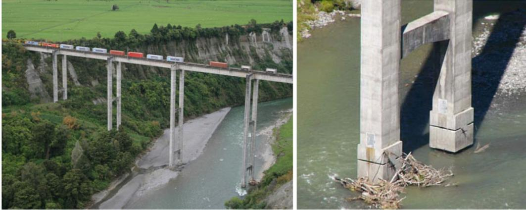
**Fig. 1** *Left* view of the South Rangitikei bridge in New Zealand. The piers are allowed to lift up to 13 cm while rocking along the transverse direction of the bridge. *Right* close view of the stepping pier at the location where uplift happens
