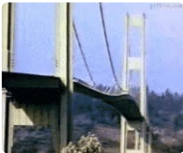
Tacoma Bridge Collapse
