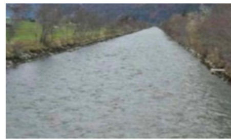
Figure 9: Channelised reach at the Hasliaare River.
